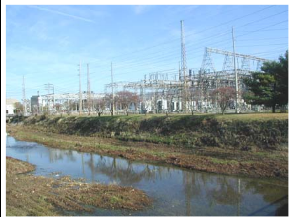
Some critical facilities, like this power substation, appear to be located without consideration of the flood or other hazard.
