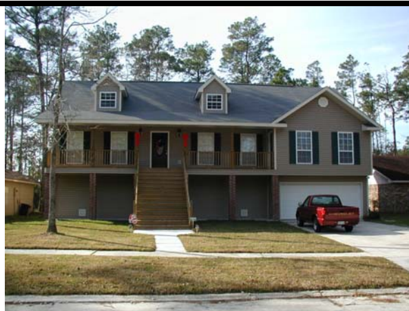
St. Tammany Parish house elevated with FEMA funding support (page 5-4)
