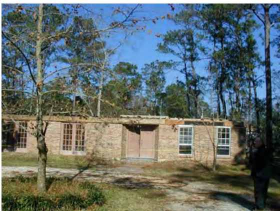
The roof has been removed as this house is being readied for a new second story.
