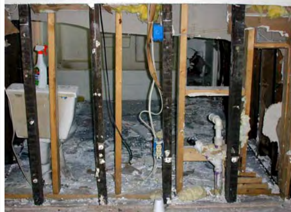
Proper cleaning after a flood requires stripping walls and floors and letting them dry thoroughly
