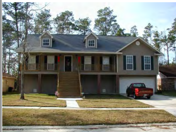
This St. Tammany Parish house was elevated with FEMA funding support.
