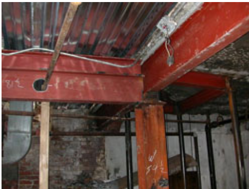
Replaced steel decking
