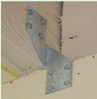
Figure 4-27. This is an example of retrofitting an existing house, originally built without hurricane clips. The popular H3 clip is used here; four nails attach the clip to the roof (truss-rafter) and four more nails attach to the wall or top plate below. For a retrofit, the clips are exposed on the outside of the house; therefore, both the clip and fasteners should be corrosion resistant and painted to blend with the exterior of the house. With the correct clip and nails you could perform the work or, if you prefer, hire a licensed contractor.
