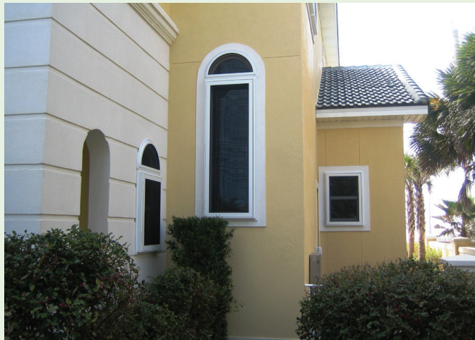
Figure 4-16. In-place stainless steel impact screen protects several windows of a coastal residence. This system requires no deployment and provides shade. Source: Roll-a-way/QMI
