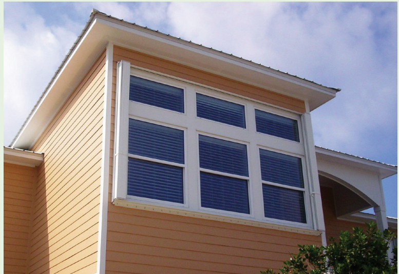
Figure 4-12. Accordion shutter (shown in the open position) installed over a large window of a coastal home. Shutter has been installed to allow deployment from inside the home. Source: Roll-a-way/QMI
