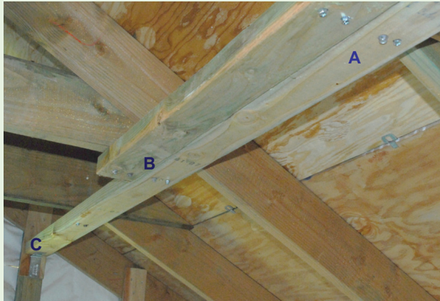
Figure 4-3. In this application of lateral bracing, the 2 x 4's are 18 inches from the ridge and connect to horizontal members that attach the opposing trusses. Not all roofs will have the horizontal members. The 2 x 4's are connected with two #14 3-inch screws (A) and overlap over two trusses (A and B). The end is connected to the gable end with an angle or L bracket (C).
