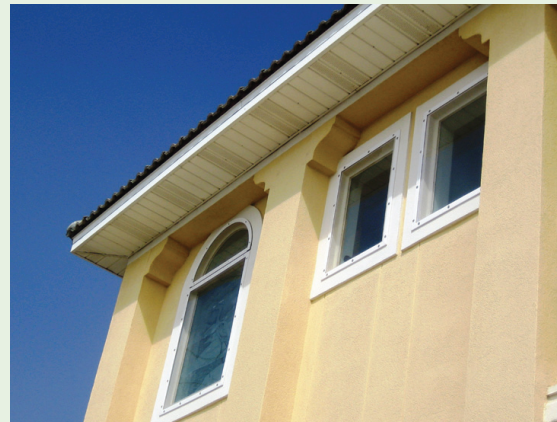
Figure 4-17. Flat impact polycarbonate panels are installed directly over windows of a coastal home. This window covering provides excellent storm protection with minimal aesthetic impact. Source: Roll-a-way/QMI
