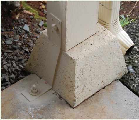
Figure 4-29. In some retrofit examples, it is possible to tie a portion of the house to the foundation. Here, a metal strap connects the vertical post to the foundation, which finishes the continuous load path connection from roof to the foundation. Source: Hurricane Protection Services.
