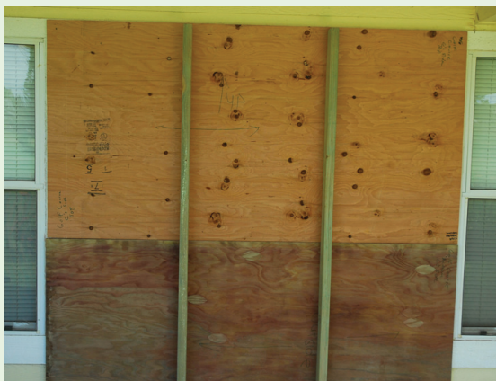
Figures 4-21 and 4-22. Not only is it necessary to install plywood opening covers correctly, it is also important to correctly label them and store them away from heat and humidity.
