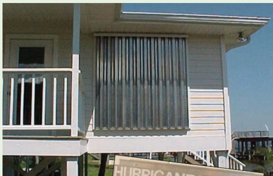
Figures 4-15. These 0.050 gauge aluminum storm panels offer cost effective storm protection. In this example, panels slip into a track above the window and secure onto a bottom track using wingnuts. Source: Roll-a-way/QMI
