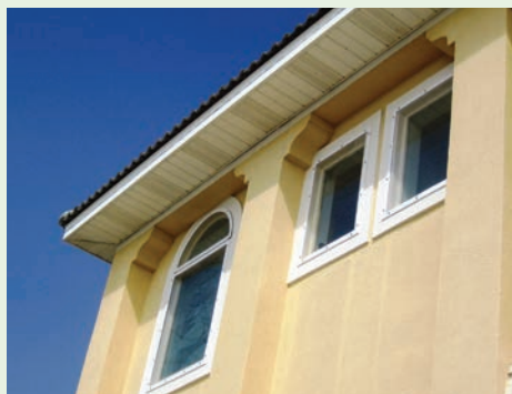
Figure 4-17. Flat impact polycarbonate panels are installed directly over windows of a coastal home. This window covering provides excellent storm protection with minimal aesthetic impact. Source: Roll-a-way/QMI
