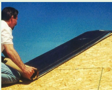
Figure 4-8. Synthetic underlayments are typically made from polypropylene, polyester or fiberglass fabric which weighs less than felt building paper, can be manufactured with anti-slip surfaces and can withstand exposure to the elements for six months. Source: Carlisle Residential
