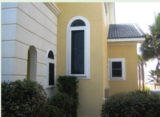
Figure 4-16. In-place stainless steel impact screen protects several windows of a coastal residence. This system requires no deployment and provides shade. Source: Roll-a-way/QMI
