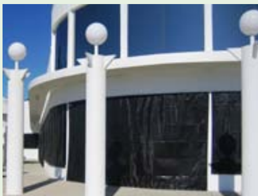
Figure 4-18. Polyethylene basketweave fabric windscreen deploys directly over ground floor windows of coastal home. Source: Roll-a-way/QMI
