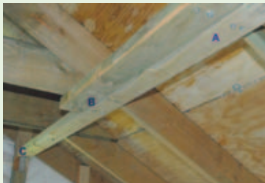
Figure 4-3. In this application of lateral bracing, the 2 x 4's are 18 inches from the ridge and connect to horizontal members that attach the opposing trusses. Not all roofs will have the horizontal members. The 2 x 4's are connected with two #14 3-inch screws (A) and overlap over two trusses (A and B). The end is connected to the gable end with an angle or L bracket (C).
